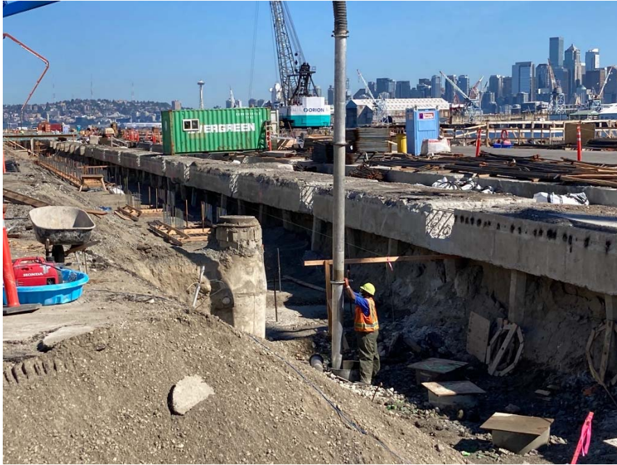
Steel Pile at Landside Crane Rail
