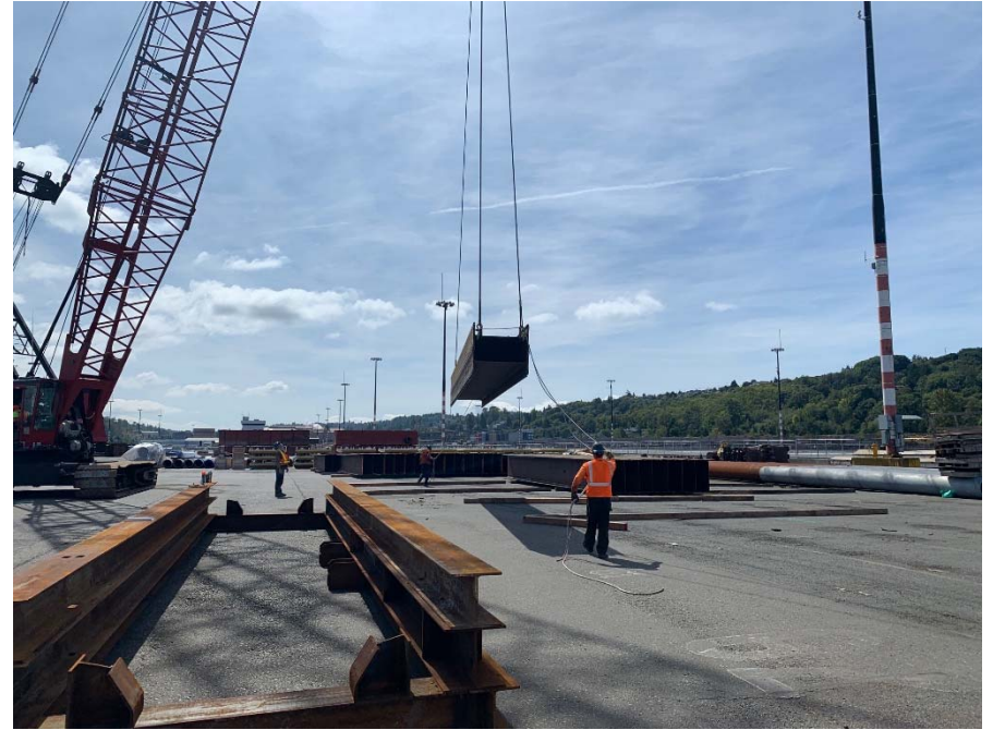
Unloading King Piles
