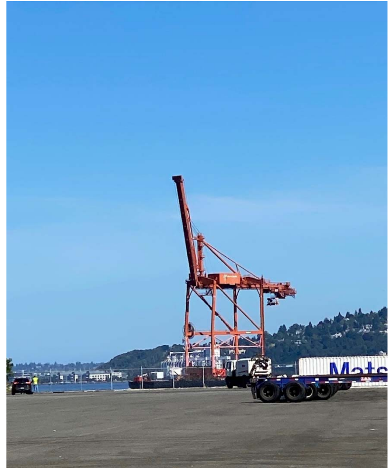
South Berth Crane Removal
