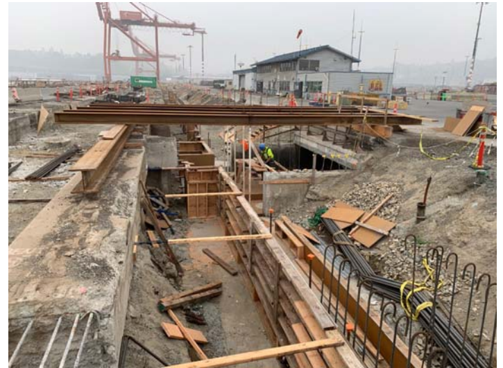
LSCR forms through conveyor tunnel
