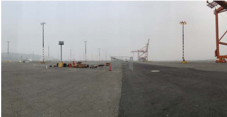
South Berth Vacant and Air Quality
